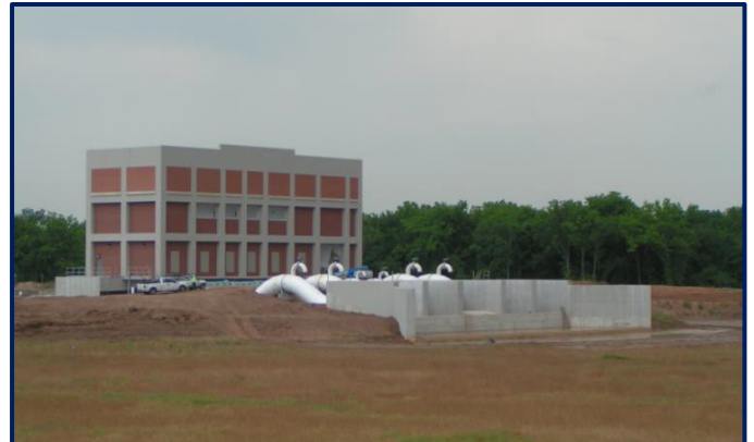
Marion Berry Pump Station, AR.
